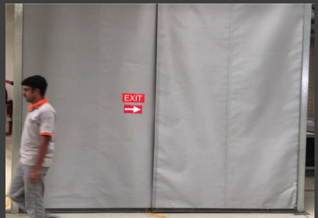
Curtain stays closed after occupants pass through
